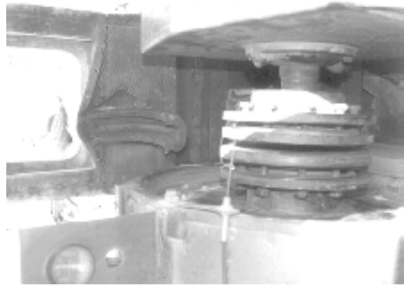
Fig.2 (Coupling of the generator and the piece of tyre lying nearby)
